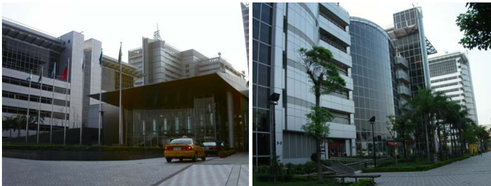
Figure 2: NKSP: the left picture shows the entrance; the right picture shows the external appearance
